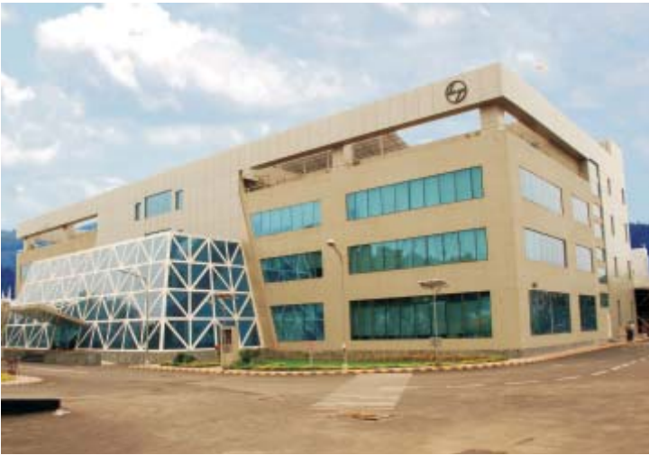
Switchgear Factory, Navi Mumbai
