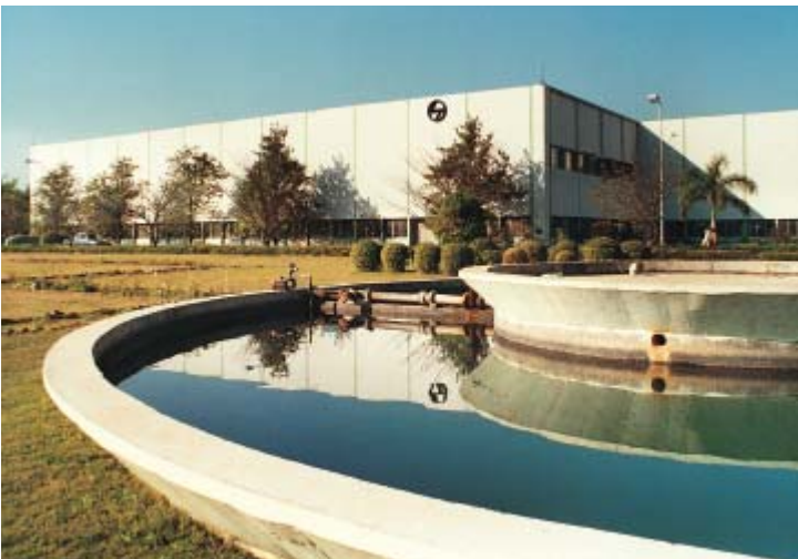
Switchgear Factory, Ahmednagar
