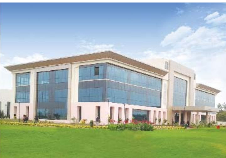
Switchgear Factory, Vadodara
